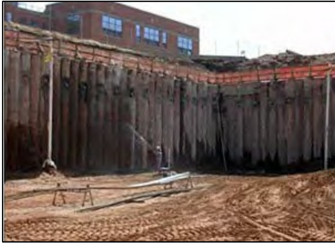
Figure 3. Secant Pile Wall.
